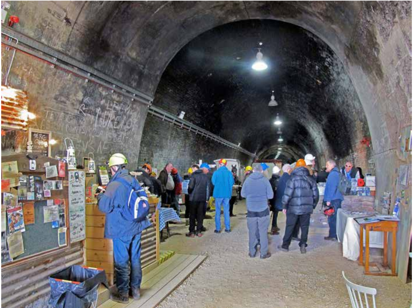
Sub Brit members gather at Ramsgate Tunnels' harbour portal at the start of the visit. Photo Clive Penfold
